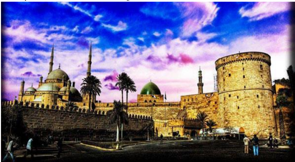
Fig. 2 The old constructions in Historic Cairo after
